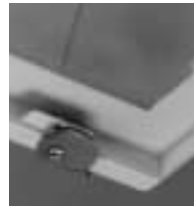
Lens silicone sealed in door frame with Dow 732 clear silicone adhesive.
